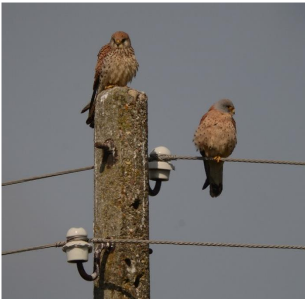
Fig. 1. Unsafe electrical pole with Lesser Kestrels.
