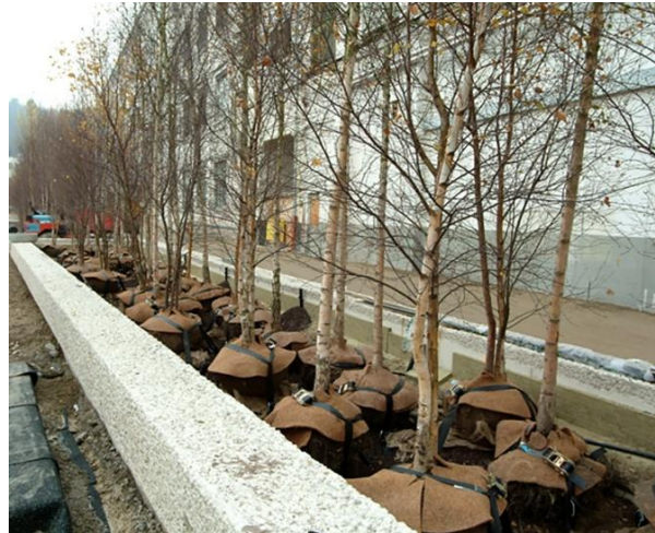
Fig. 5. Systems for underground anchoring of newly planted trees – stripe of high-density trees ( https://www.greenmax.eu/de/wurzelballenverankerung/ )
